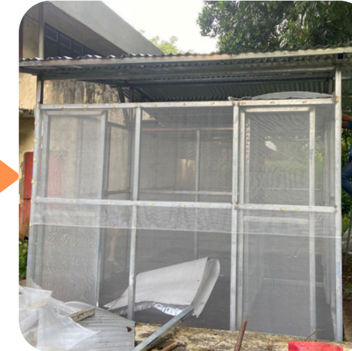
Establishment of Facility
